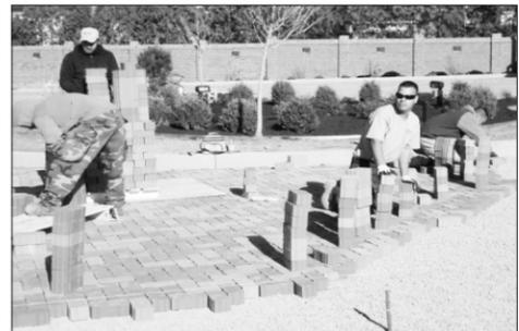
Pavers were laid by hand over an 18" gravel bed.
